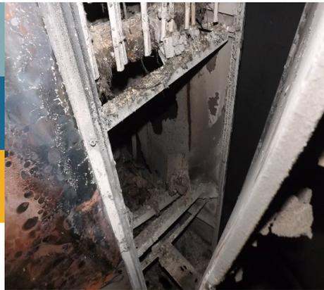
*An arc flash is a powerful energy release. Even metals can melt and evaporate in the high temperatures.*
