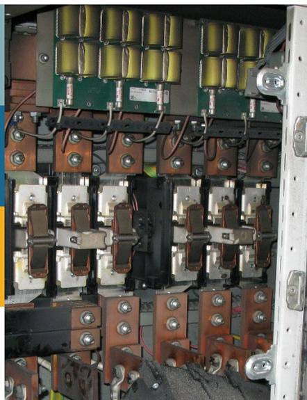
*Soot in high voltage installations can cause arc flashes as the soot is conductive.*
